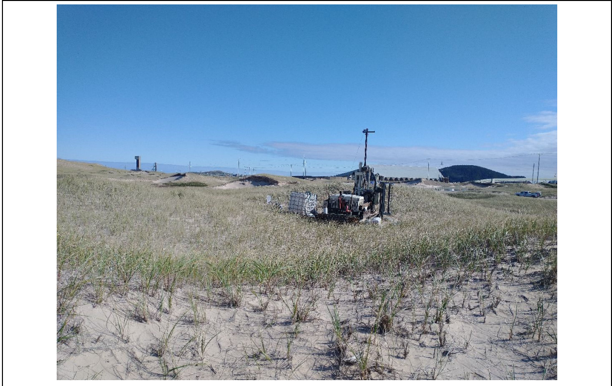
Figure 4 Site du forage F-03
