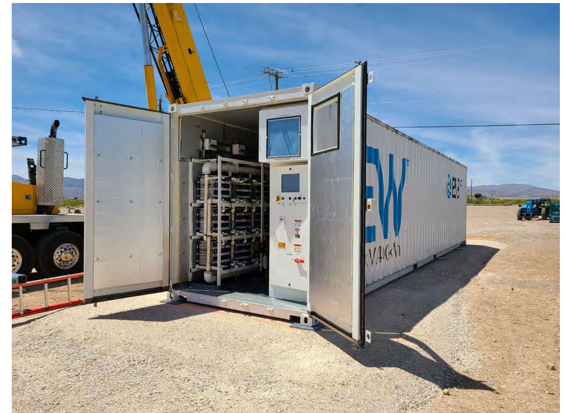
Exemple d'installation de batteries de stockage / Example of a storage battery installation, © Photo ESS Tech
