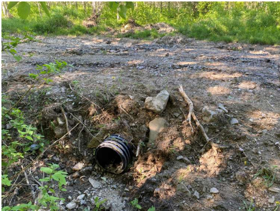
6. Ponceau CE-15, aval
