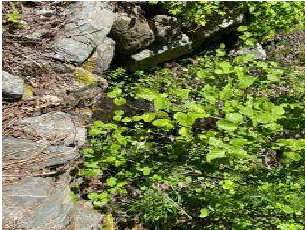
36. Ponceau CE-51, aval
