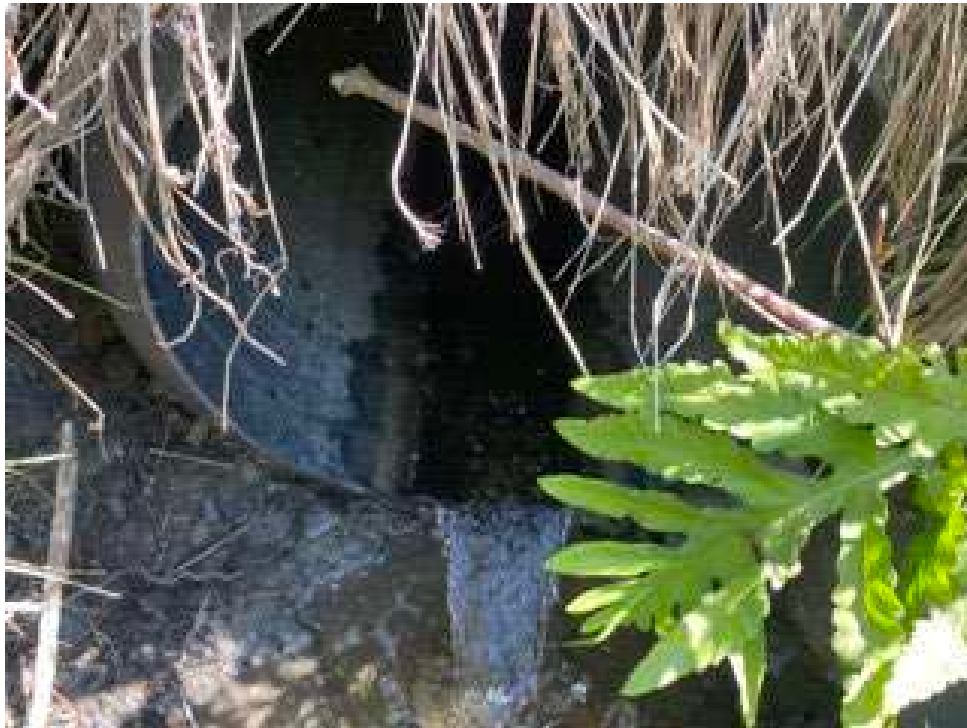
34. Ponceau CE-50, aval
