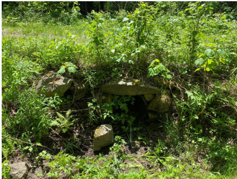
12. Ponceau CE-30, aval
