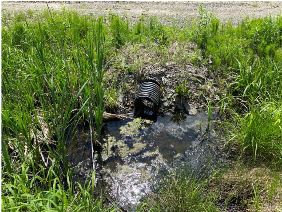
14. Ponceau CE-31, aval
