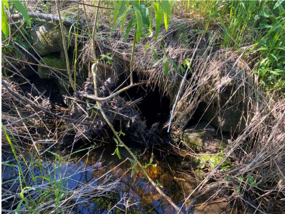
3. Ponceau CE-13, amont
