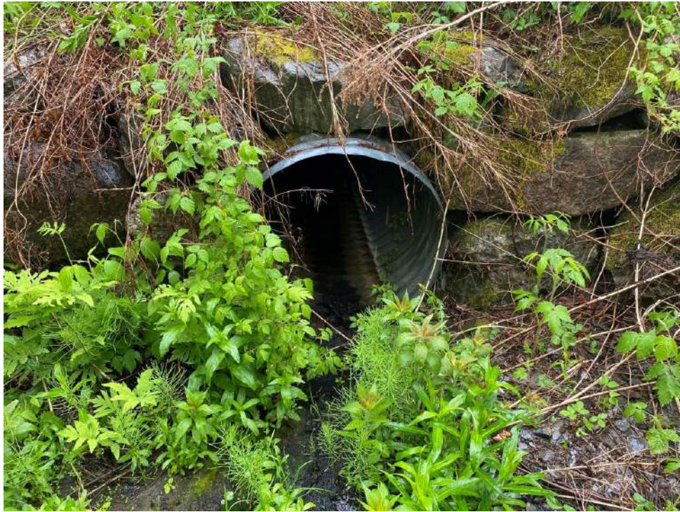
37. Ponceau CE-54, amont
