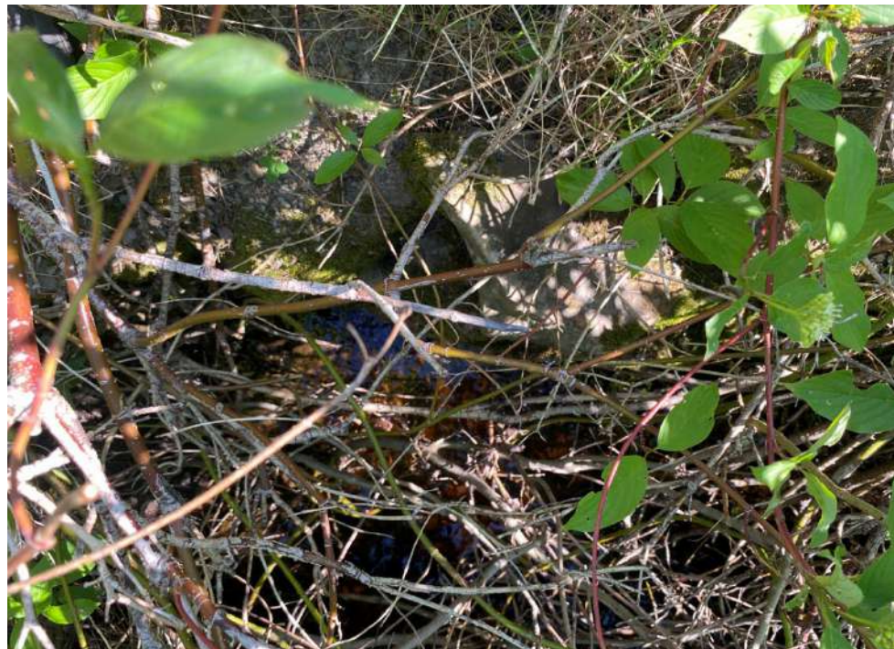
4. Ponceau CE-13, aval
