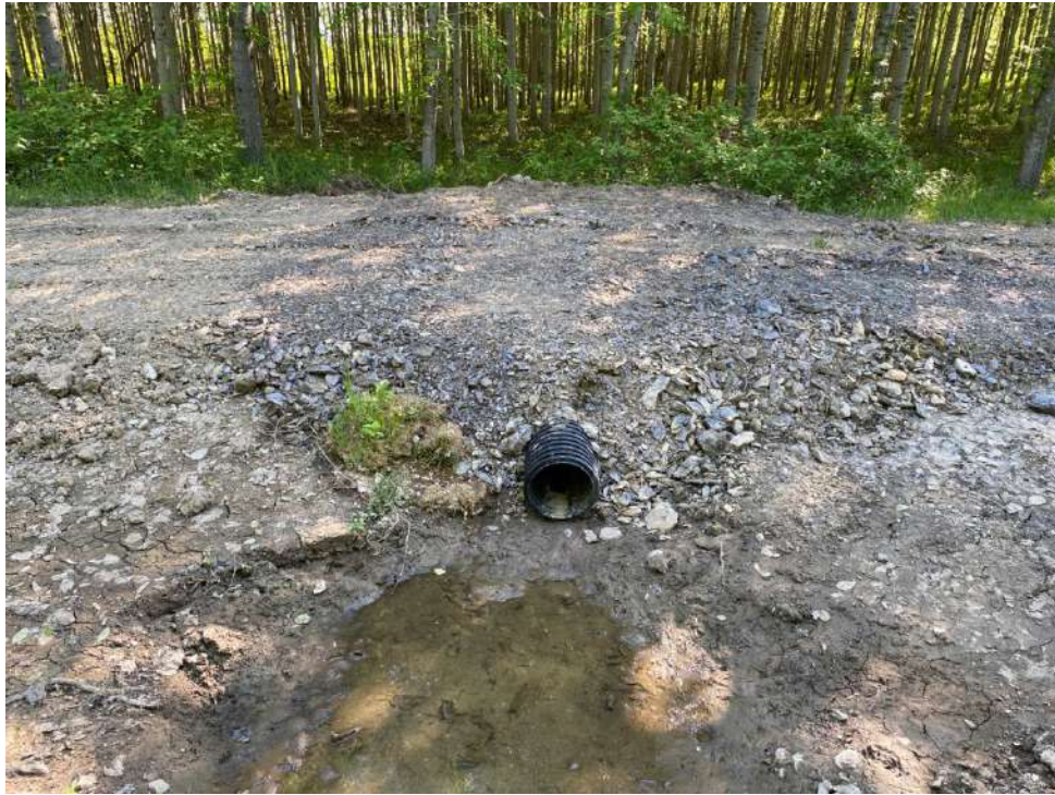
5. Ponceau CE-15, amont
