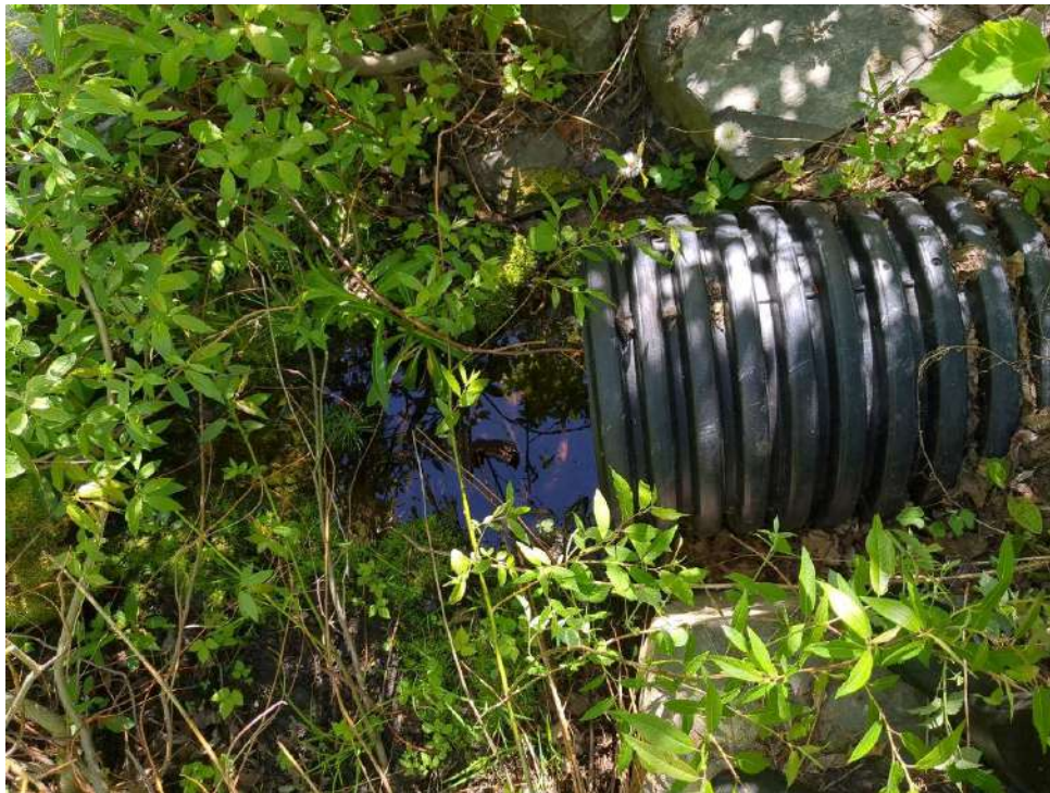
39. Ponceau CE-55, aval
