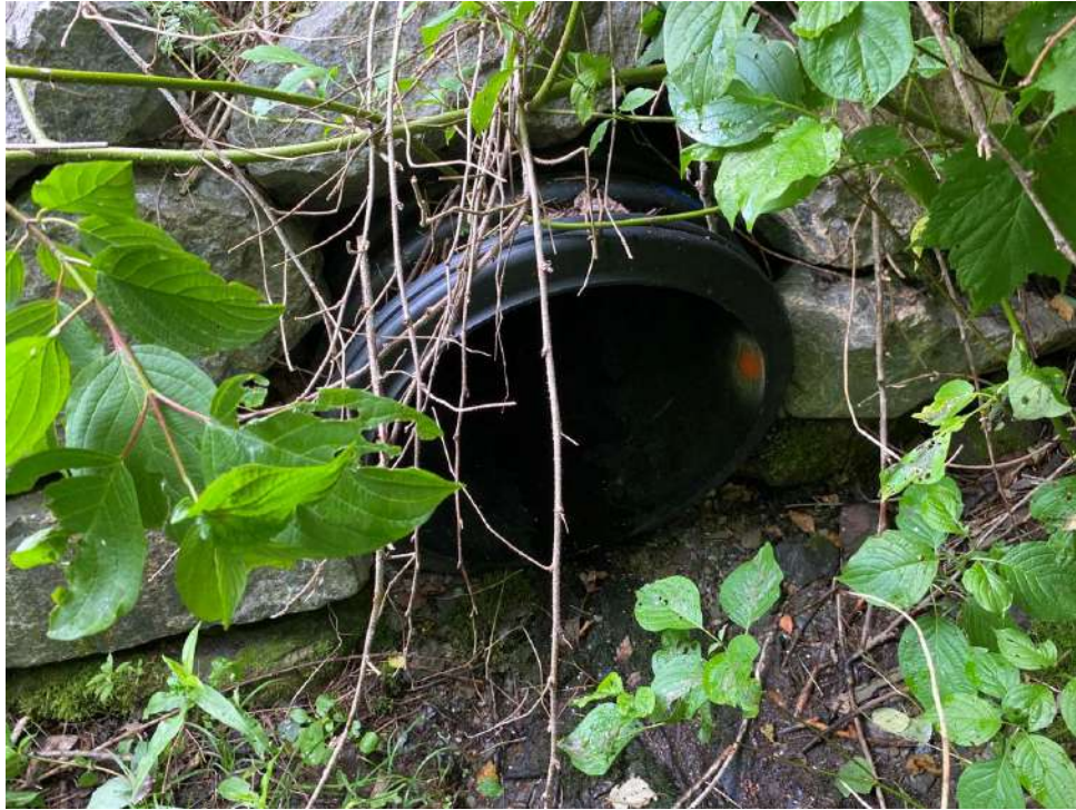
43. Ponceau CE-58, aval
