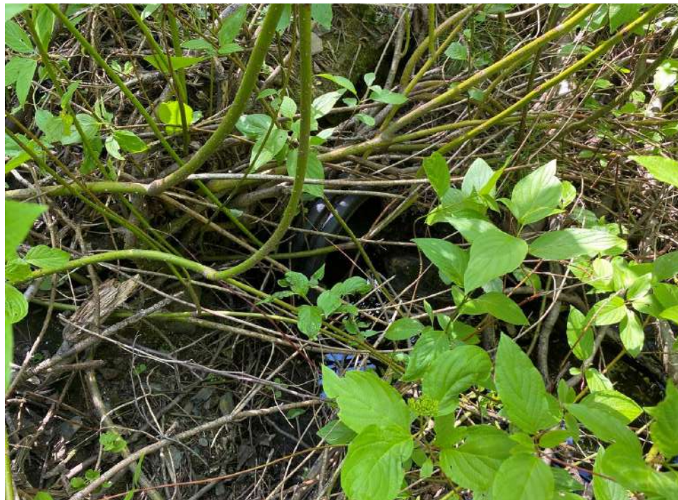
16. Ponceau CE-33, aval
