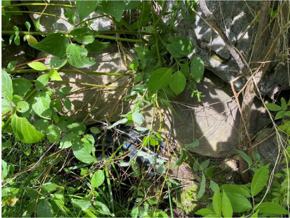
41. Ponceau CE-57, aval
