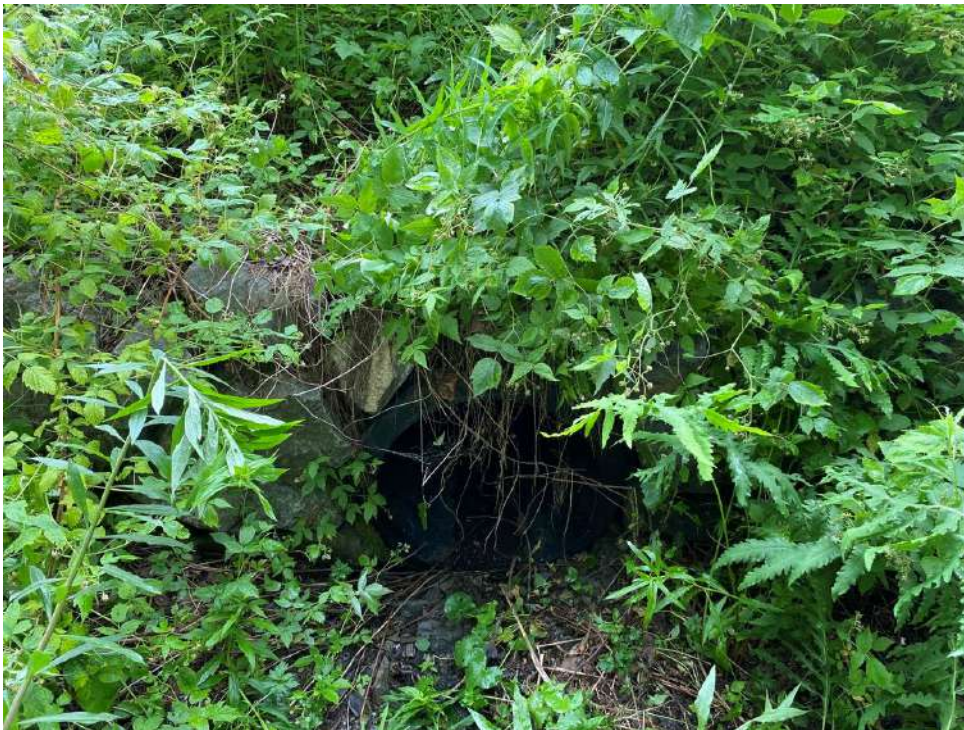
42. Ponceau CE-58, amont
