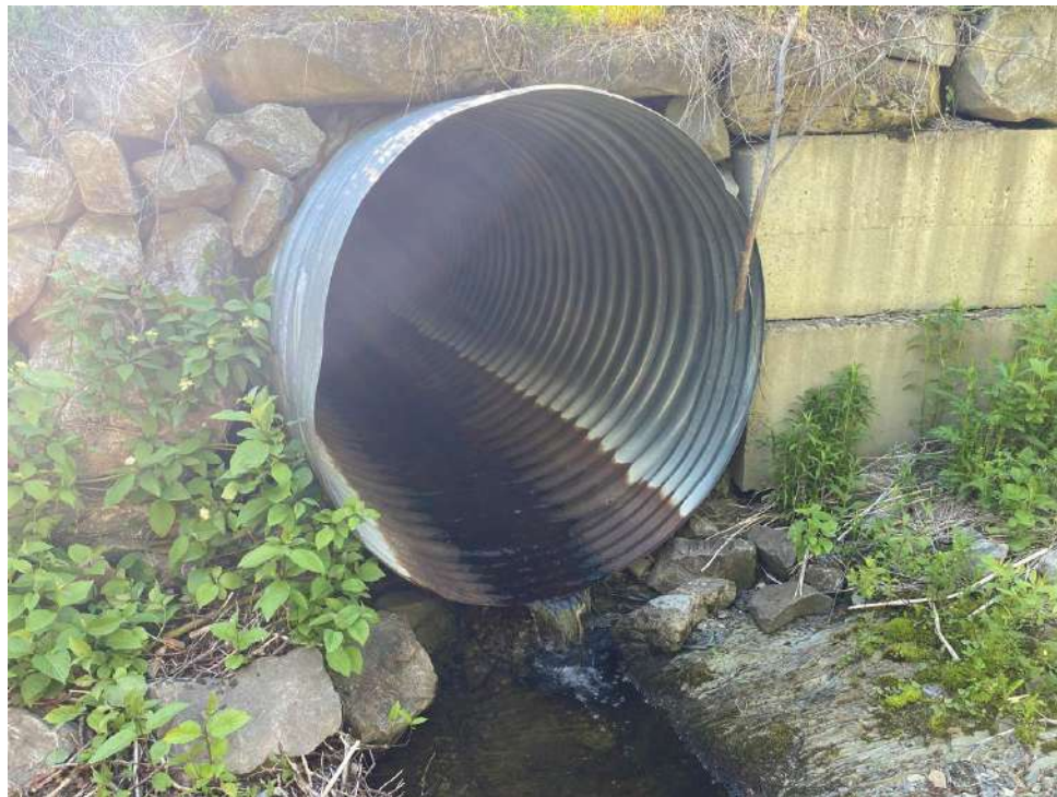
32. Ponceau CE-48, aval
