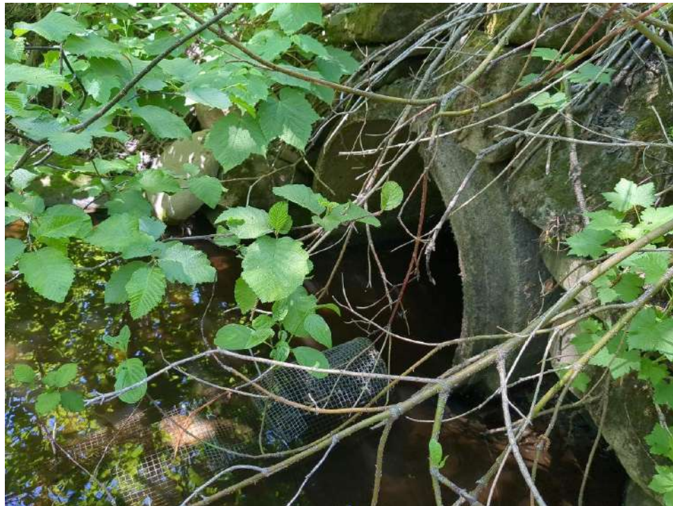
8. Ponceau CE-19, aval
