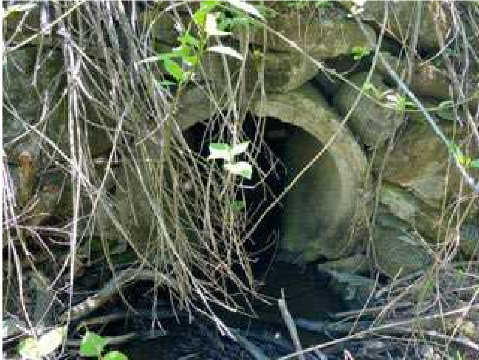
7. Ponceau CE-19, amont
