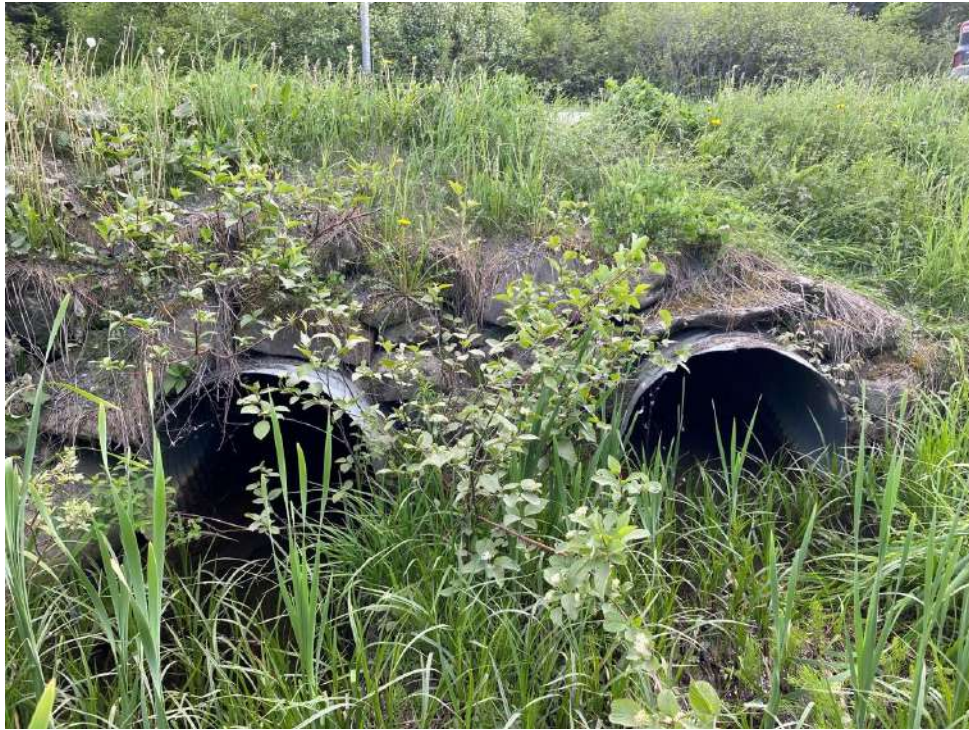
17. Ponceau CE-34, amont
