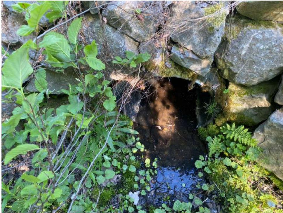
35. Ponceau CE-51, amont
