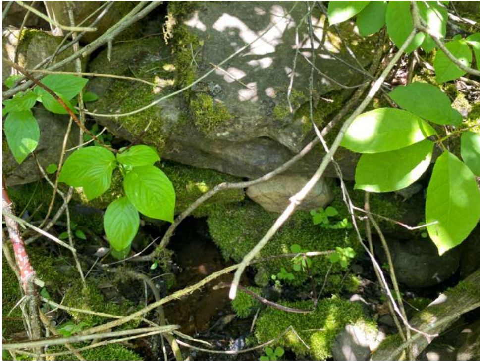
33. Ponceau CE-50, amont
