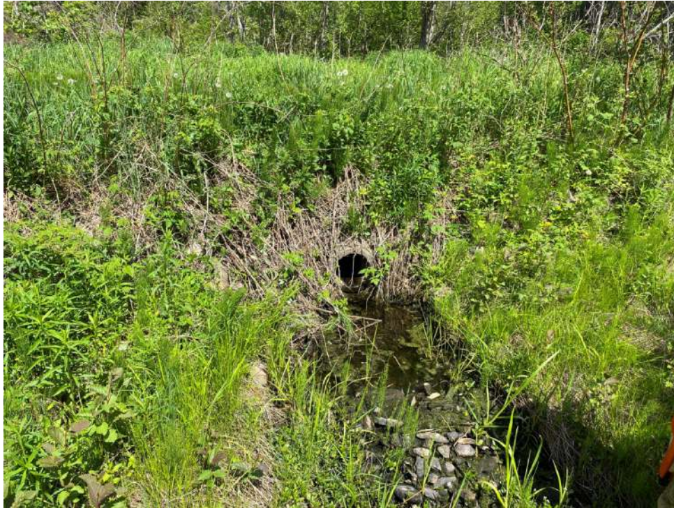
13. Ponceau CE-31, amont
