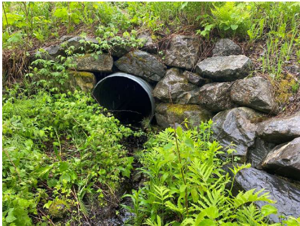
38. Ponceau CE-54, aval
