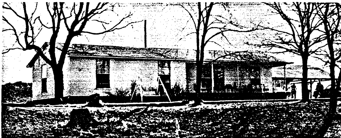
Figure 19.—Test structure 23, near a quarry.
