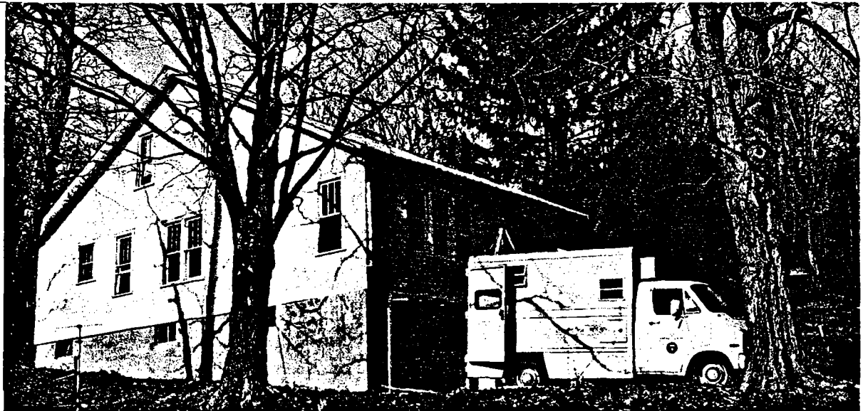
Figure 26.—Test structure 49, near a coal mine.
