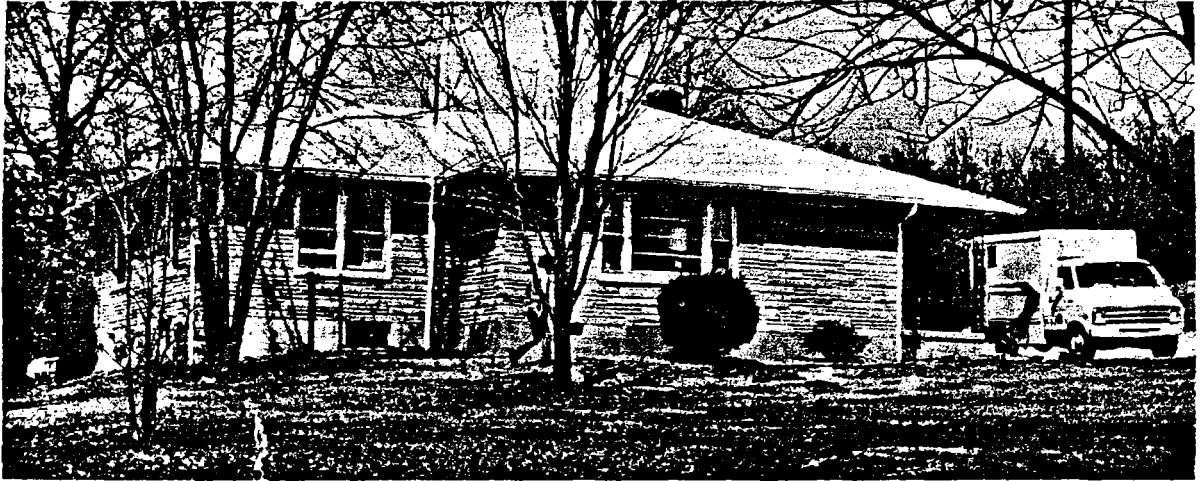
Figure 24.—Test structure 30, near a coal mine.
