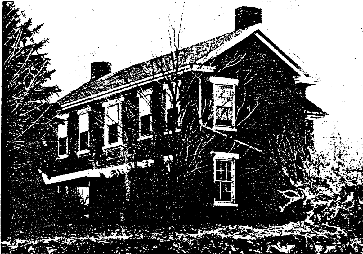
Figure 27.—Test structure 51, near a coal mine.
