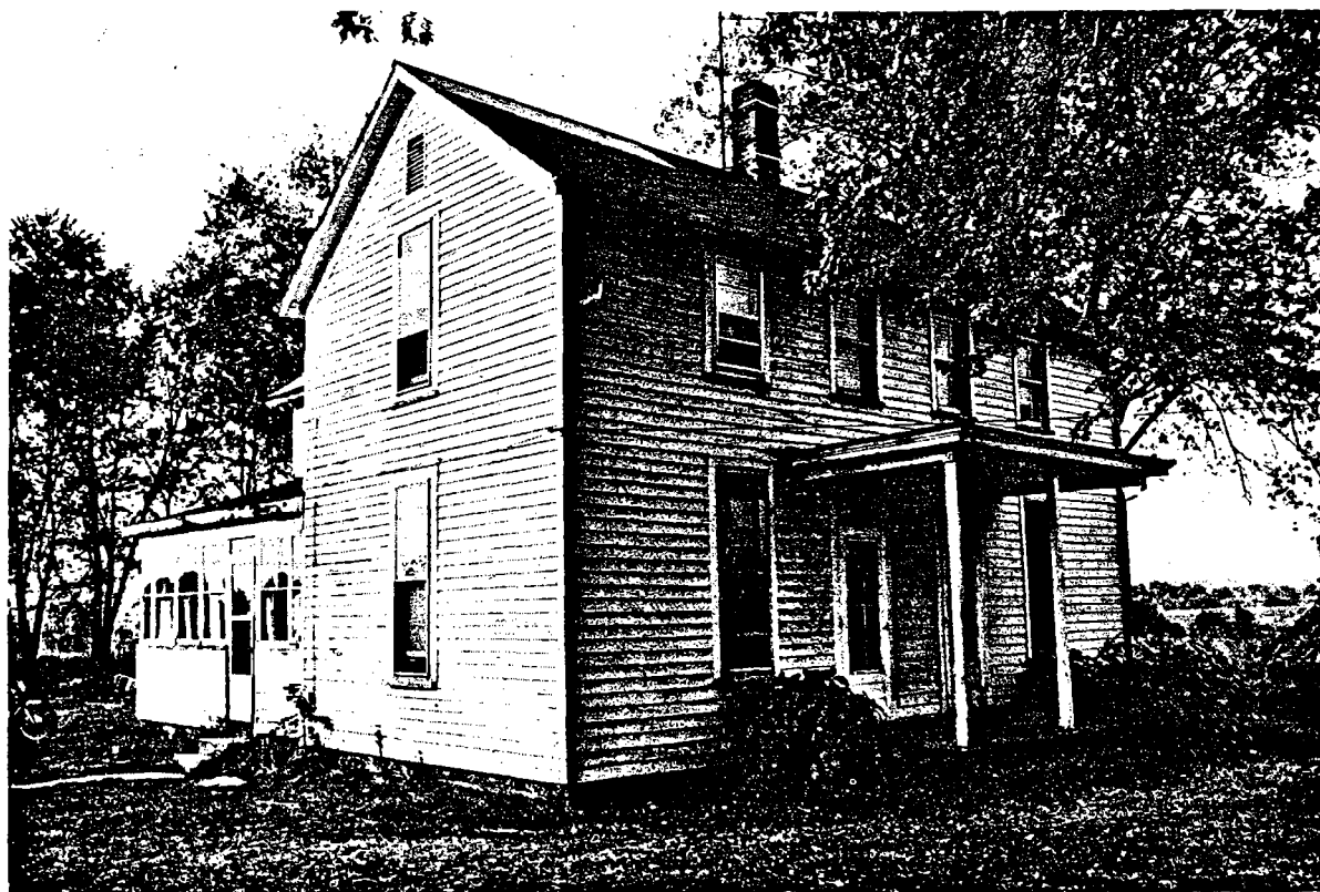
Figure 15.—Test structure 19, near a coal mine.
