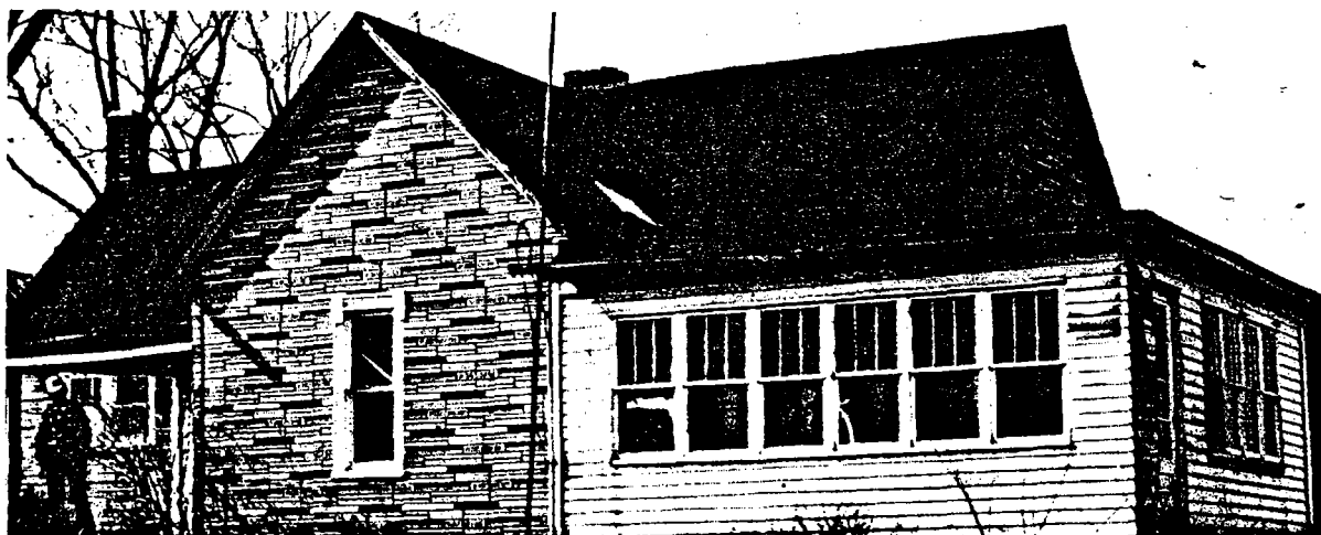
Figure 21.—Test structure 27, near a coal mine.
