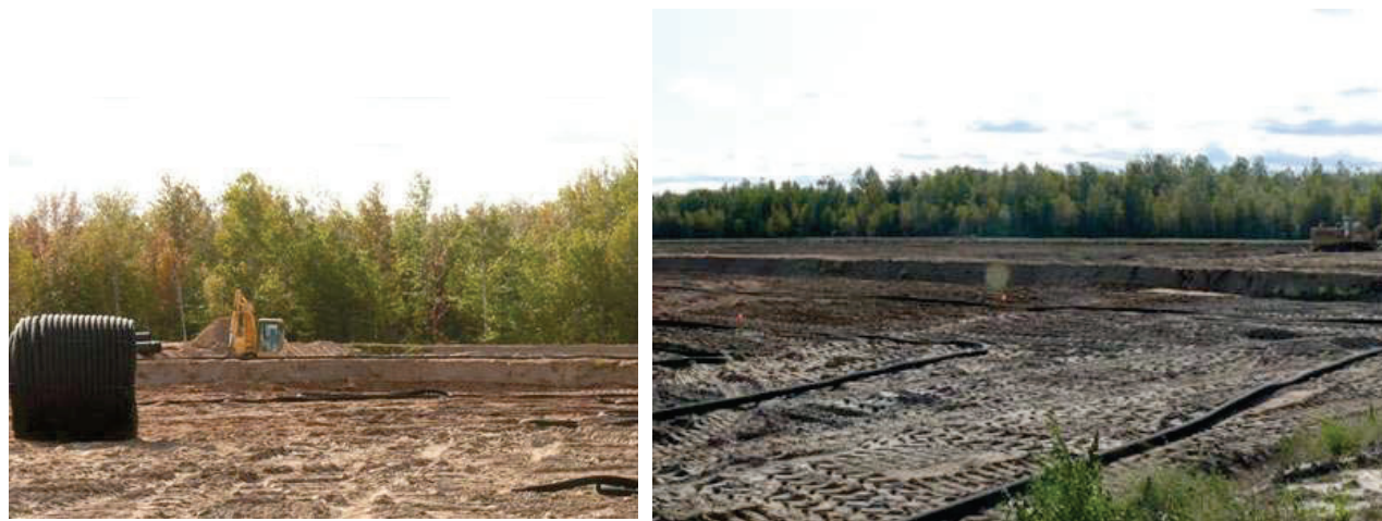
Figure 7. Installation des drains
