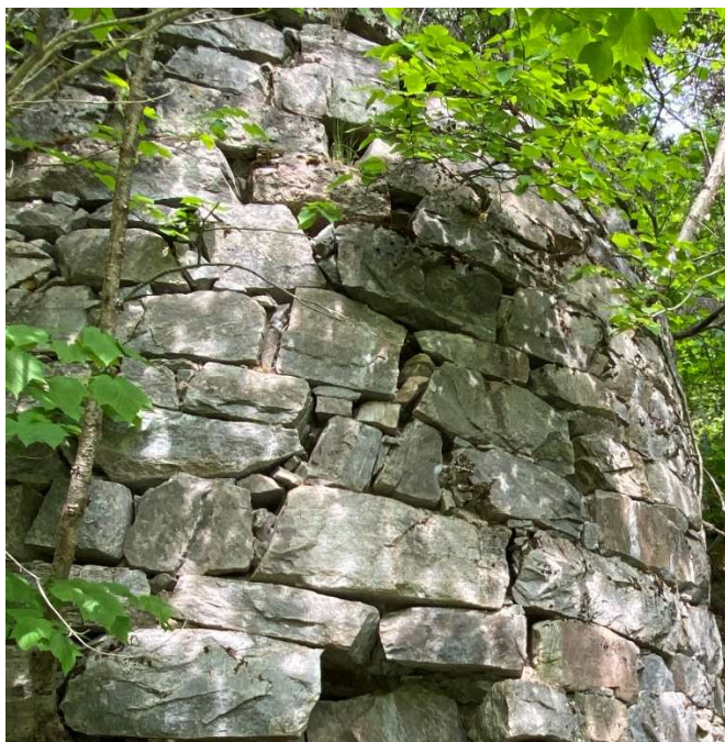
Figure 6 : Appareillage assisé. Elizabeth Cloutier © CCQ (MCC), 2023.
