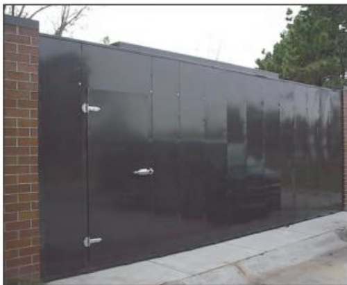
Air-cooled chiller attenuation systems
