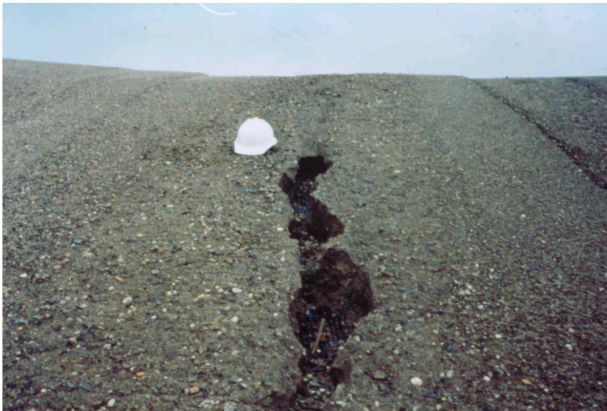
Figure F-A.2.1. Construction debris in a CCL with an initially smooth surface protruded from the CCL after the CCL was left exposed and subsequently eroded.
