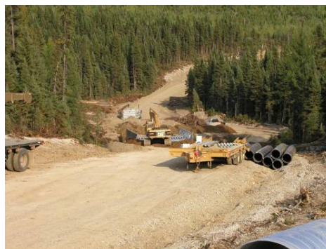
Construction de chemins forestiers
