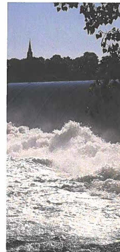
Barrage de Chambly.
