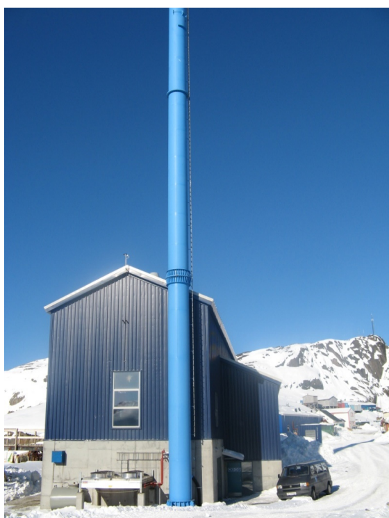
Picture 1: Example of 400 kg/h WtE facility – Maniitsoq
