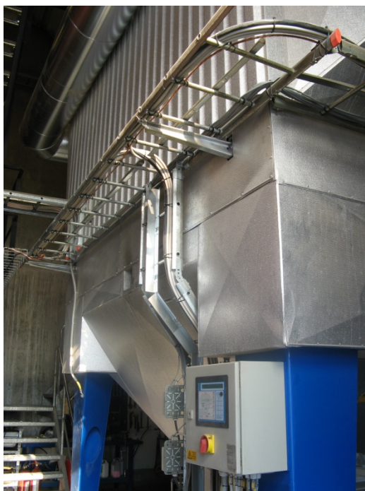
Picture 5 - View of the ESP
