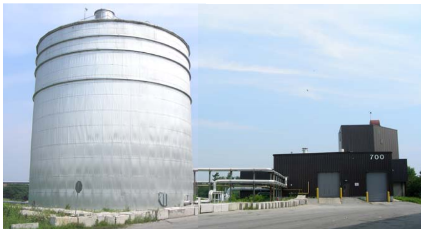
Figure 5.6 Dufferin Organics Processing Facility à Toronto (Photo : SOLINOV)
