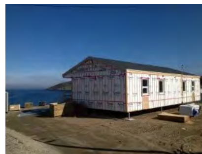
Figure 5: Housing construction Source: Makivik Construction
