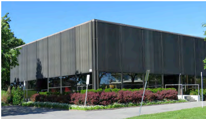
Station de pompage du parc Roland-Beaudin. 929, avenue Roland-Beaudin.
