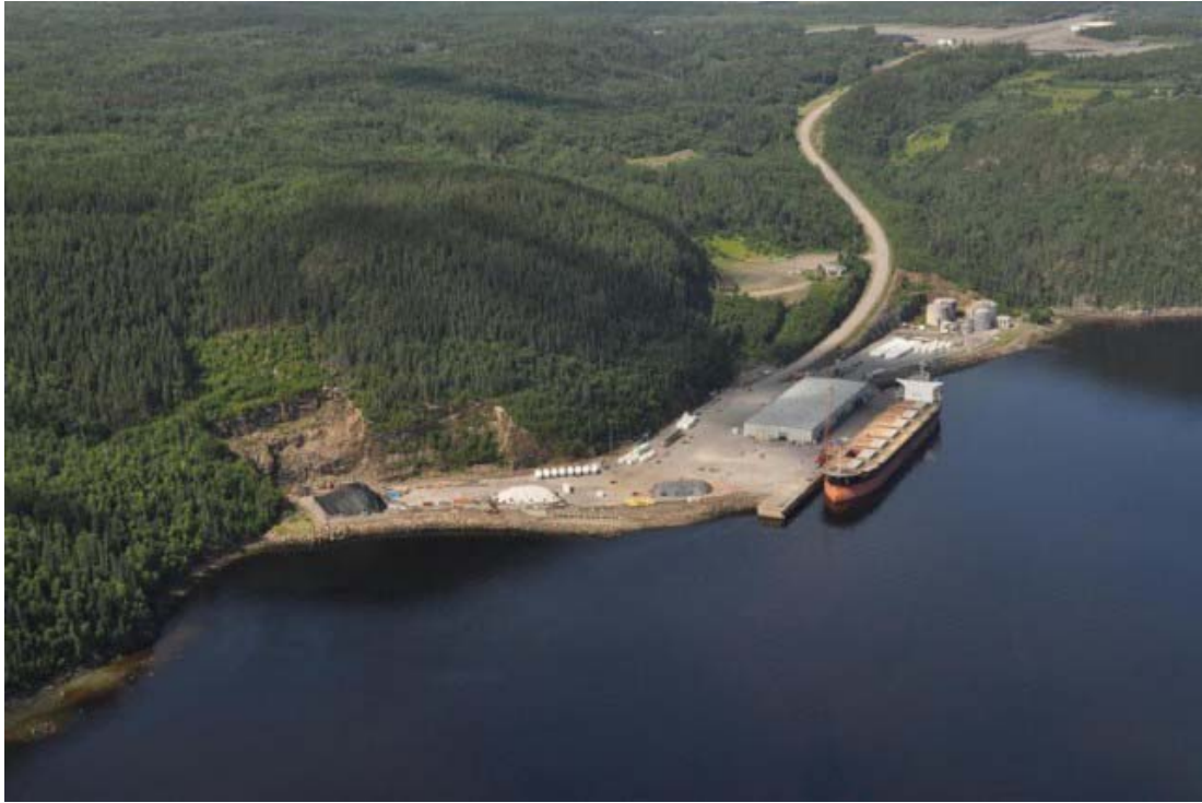
Figure 49 Terminal maritime de Grande Anse
