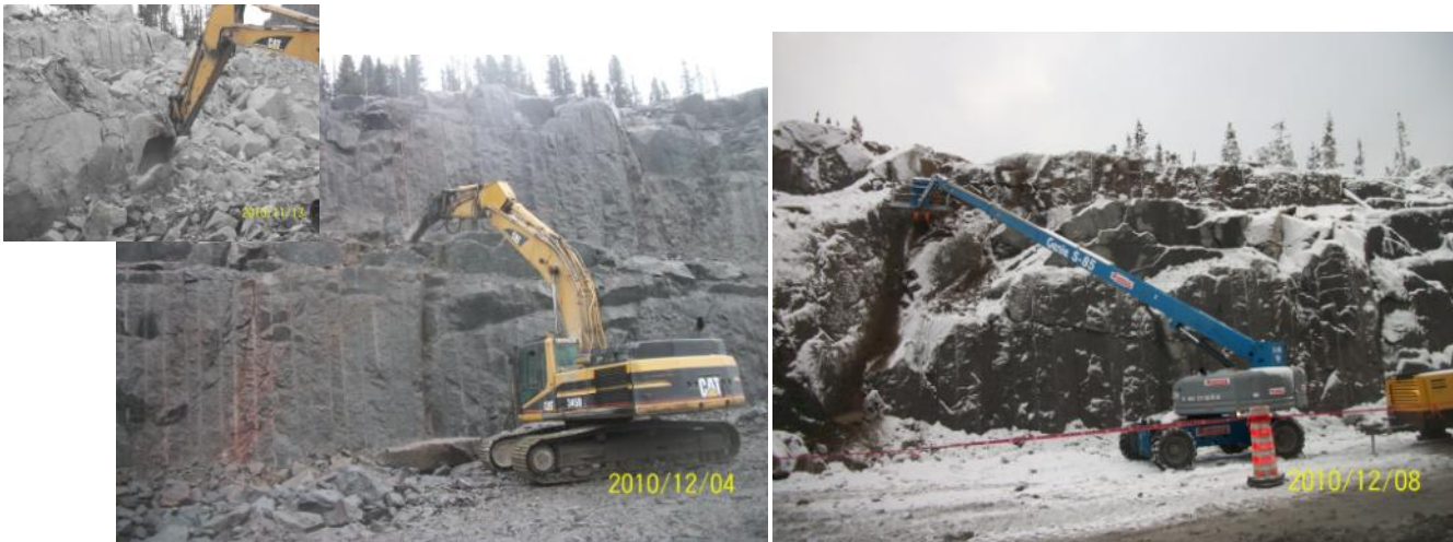
Figure 10-2: Scaling methods; (left) using excavator (right) using a lift and steel bars to pry loose rocks off.
