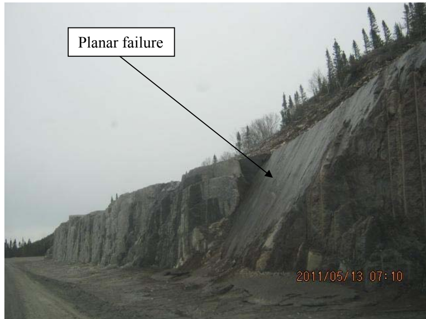
Figure 9-1: Planar failure in a rock wall.
