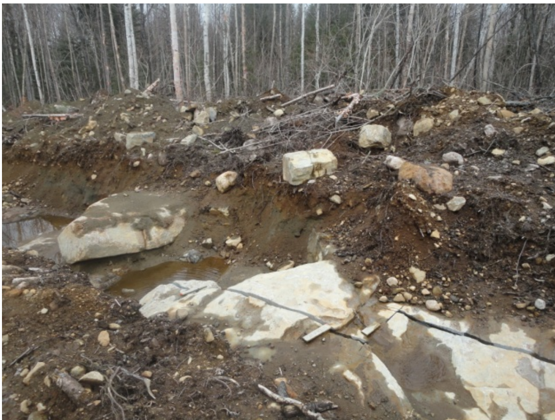
Figure 6-4: Overburden Encountered on Tony Block Site
