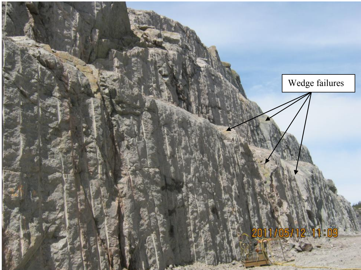
Figure 10-1: Pre-shearing blast over three 15 m high benches.
