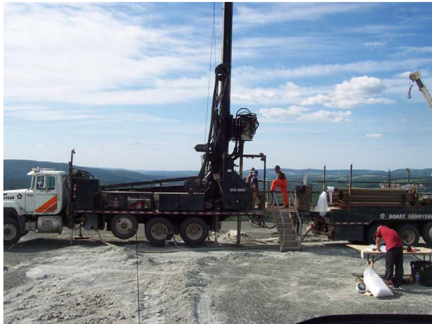
Figure 9: Sonic Drilling set-up at NOR-1 drill hole on the Normandie tailings pile.
