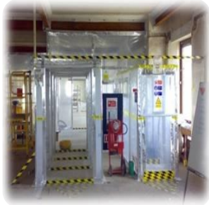
Designated work area
