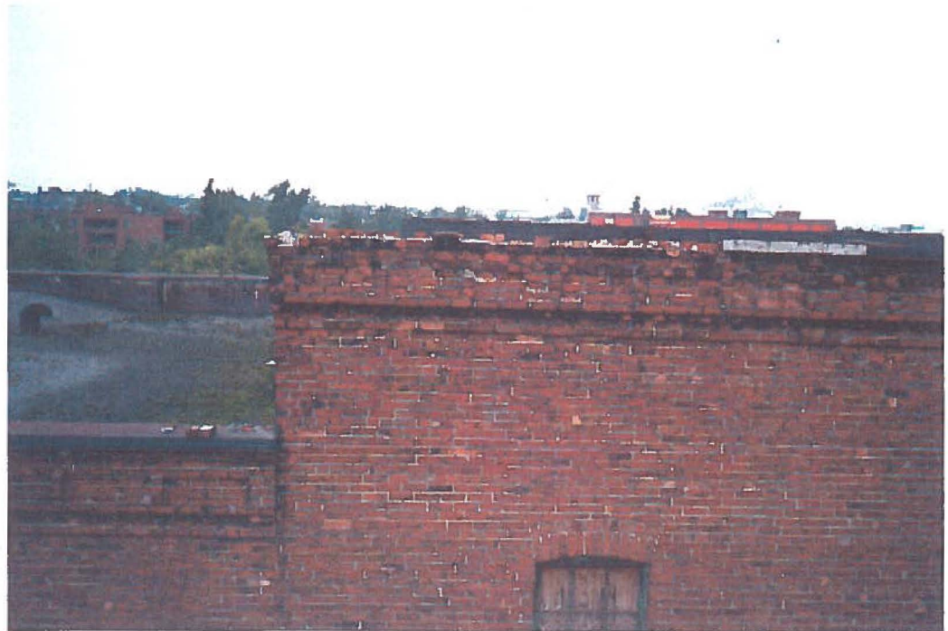
Photo 4: Parapet: section A - Mur Ouest.
